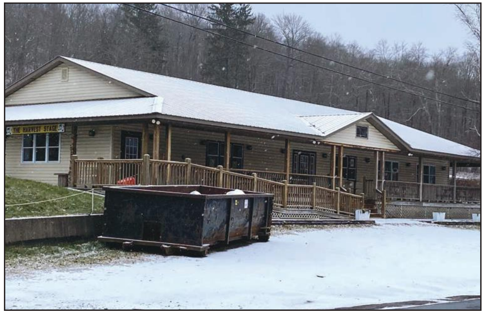
A dumpster was brought for the cleanout of the Catskills Regional Harvest building on Route 28, Andes after the shop was closed last fall. The closing of the business has resulted in losses for vendors taxpayers.
