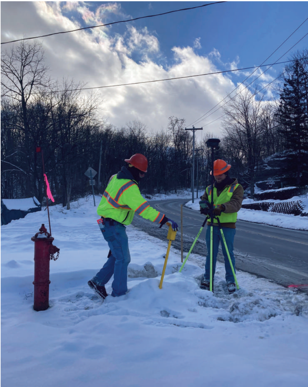
A survey crew was spotted on Main Street in Village of Sharon Springs on Wednesday (2/1) afternoon taking measurements for sidewalks, particularly "ADA Compliance and correcting corners" in relation to the multi-step Water & Sewer Project.
