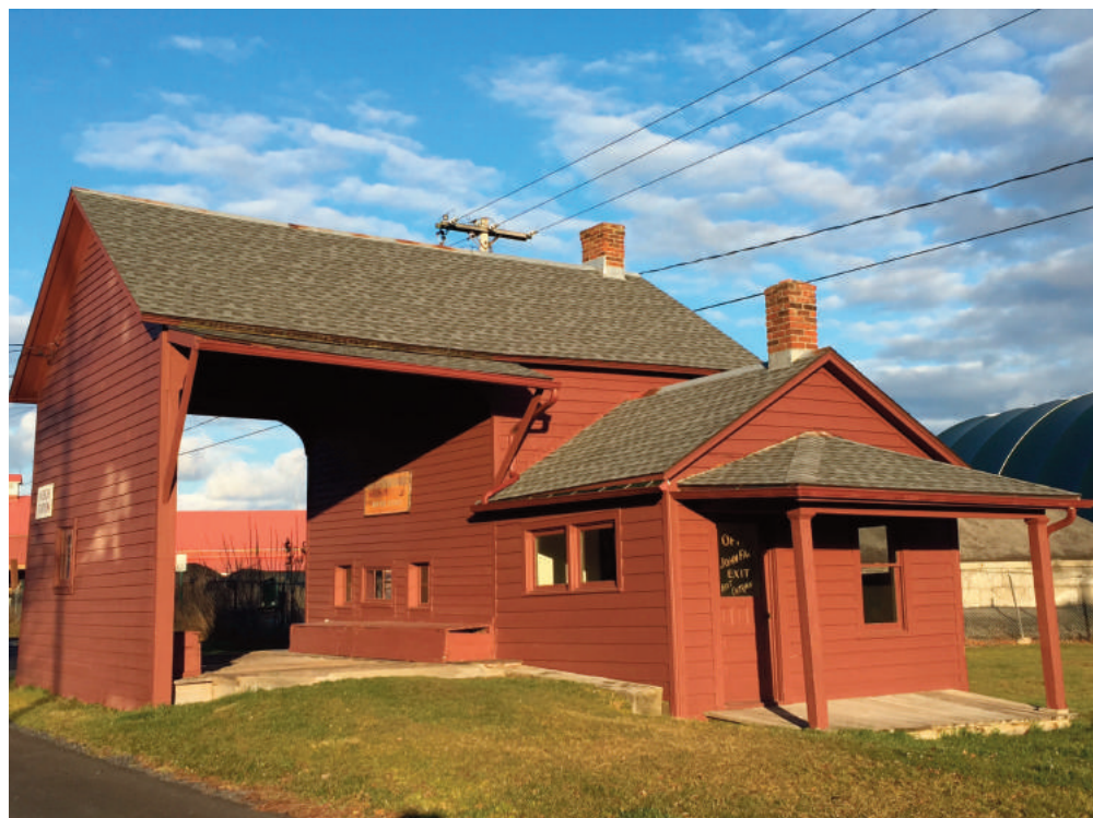
The new roof on the weigh station.
