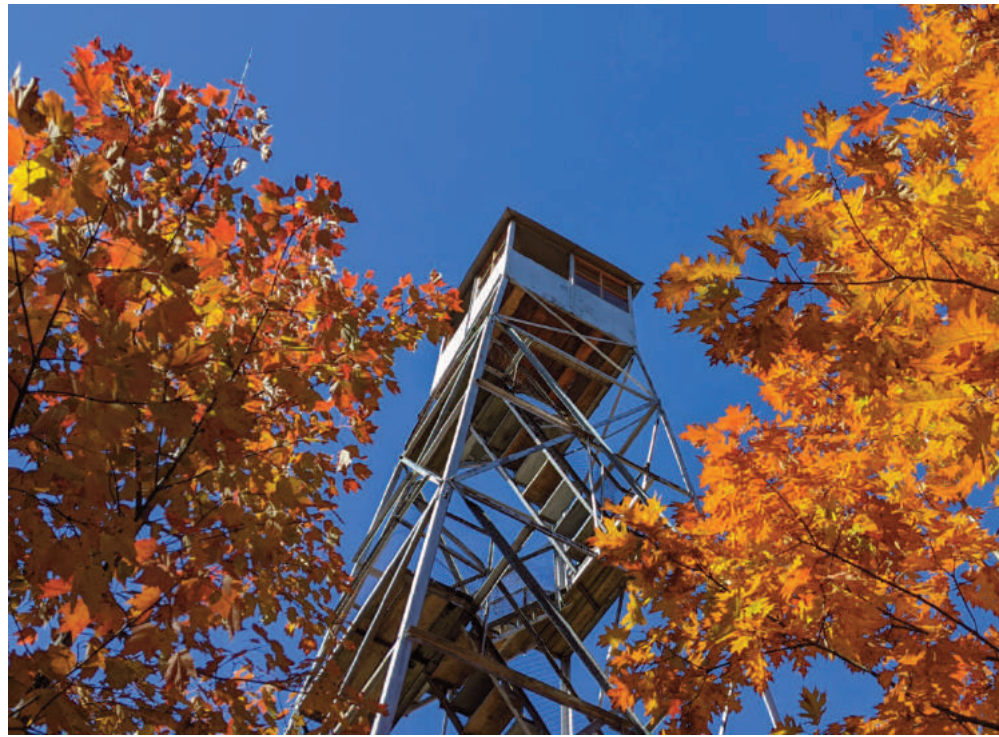
One of six fire towers located on the peaks of the Catskill Mountains. Photo courtesy Gary Keir.
